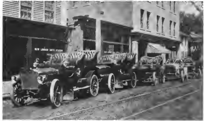
NEW GARAGE OF C. K. SMITH AT NEW LONDON
